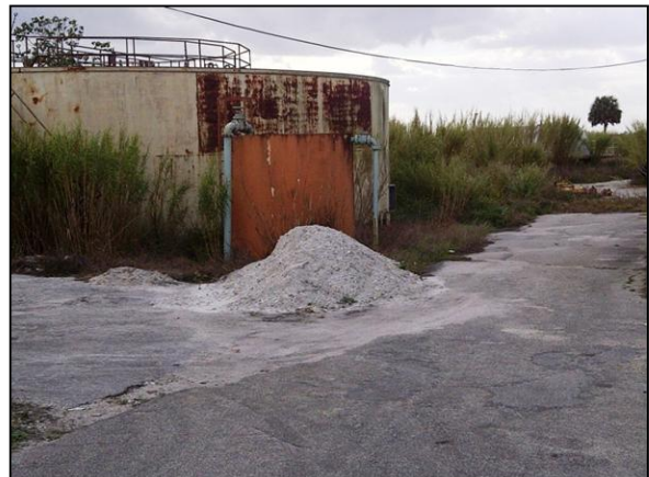
Waste Water Treatment Plant: Clean-Up
