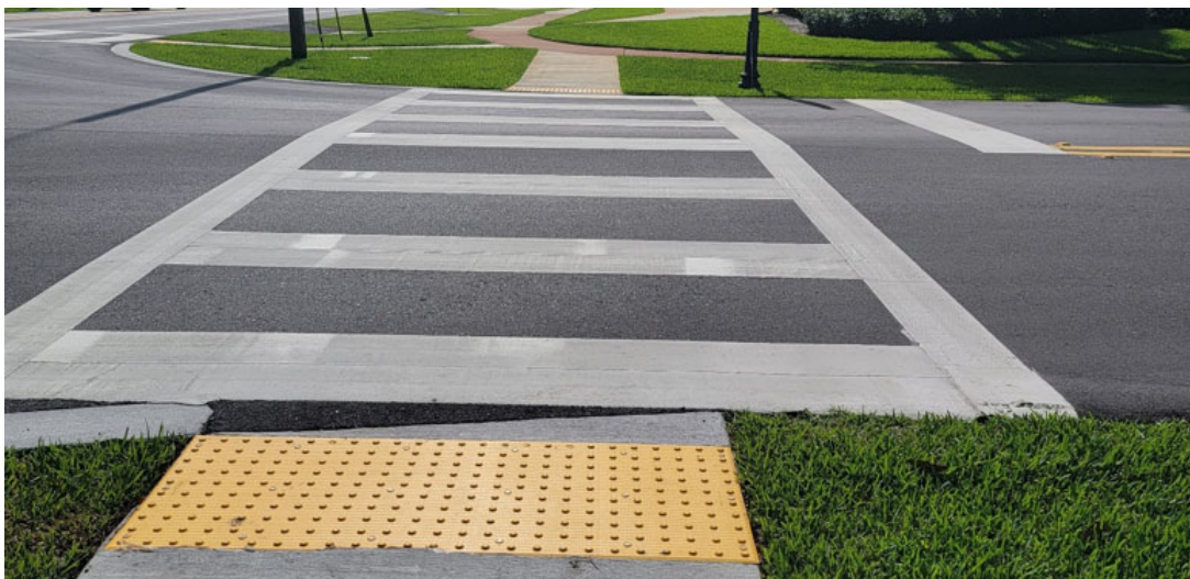
Photo taken on 5-23-22 of a section of the Header Curb at the Lighthouse/Anchorage Intersection
