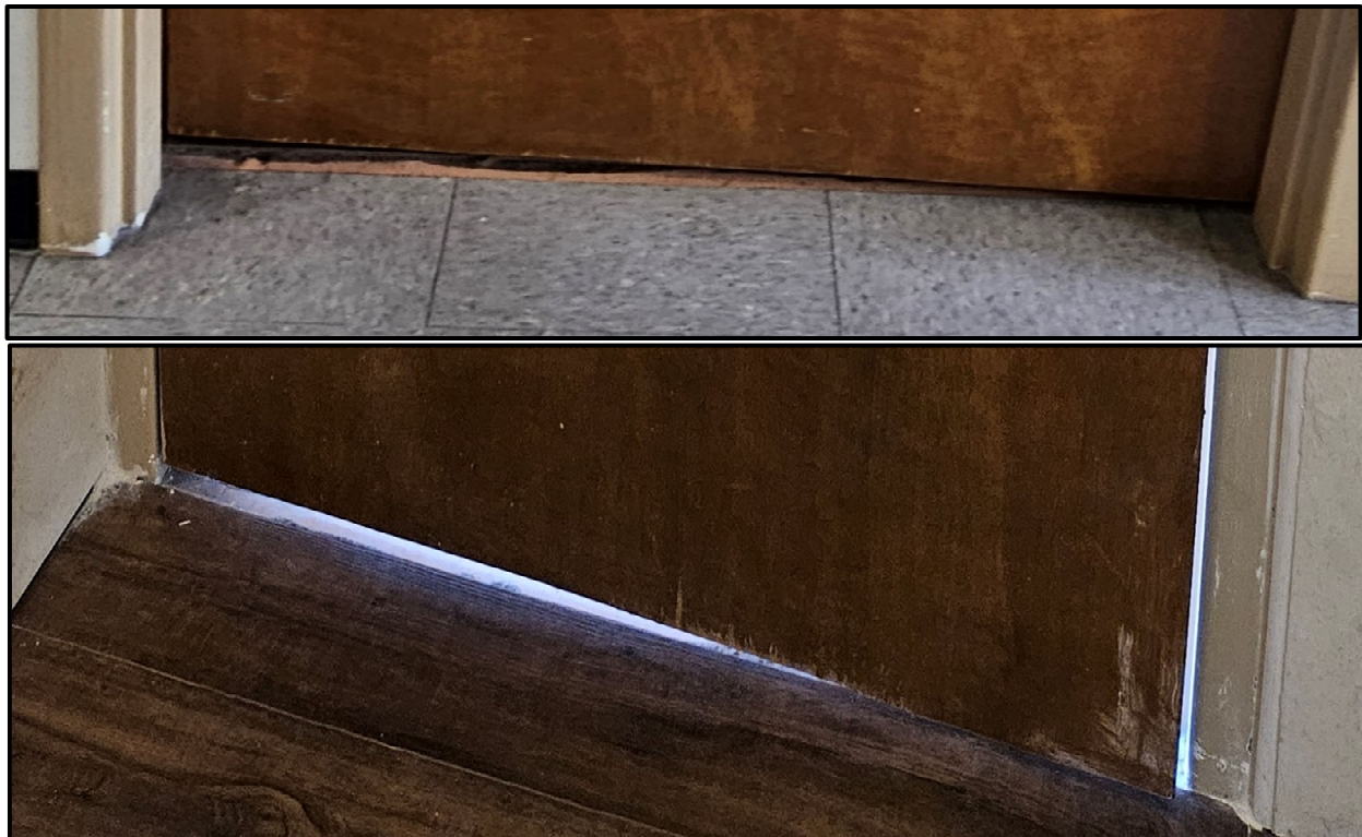
4. Poorly fitting entry door (shown from outside and inside):
